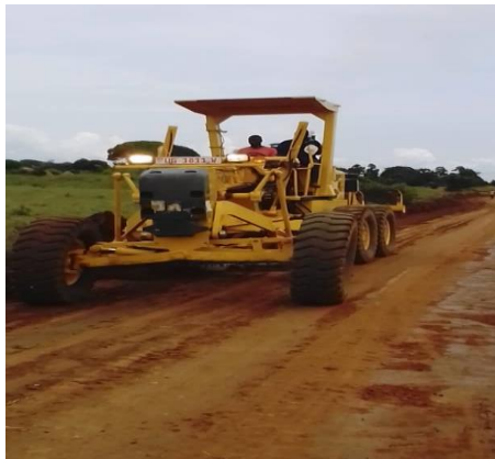
Mechanized Road Grading and Repair using District Equipment
